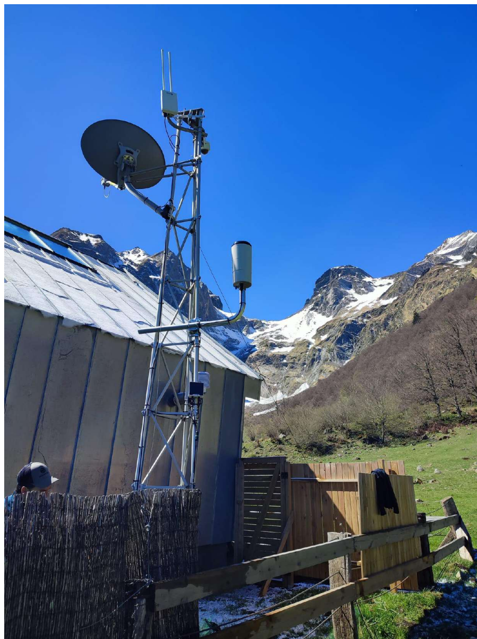
Figure 4. Installation of device.
